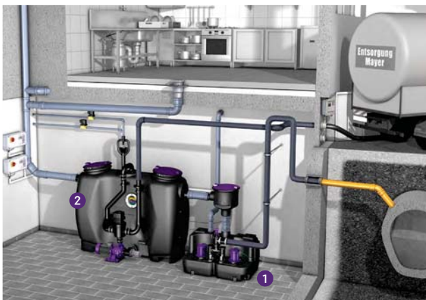
1 Lifting station 2 Grease separator EasyClean
