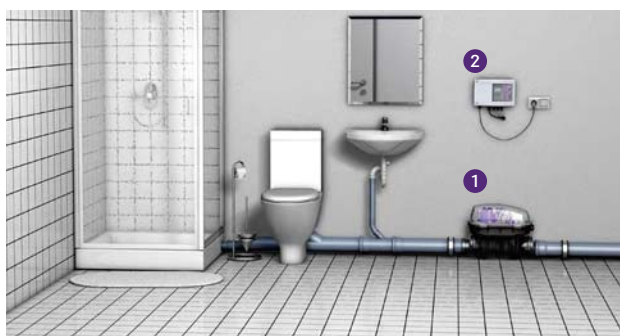
1 Backwater pumping station 2 Control unit
