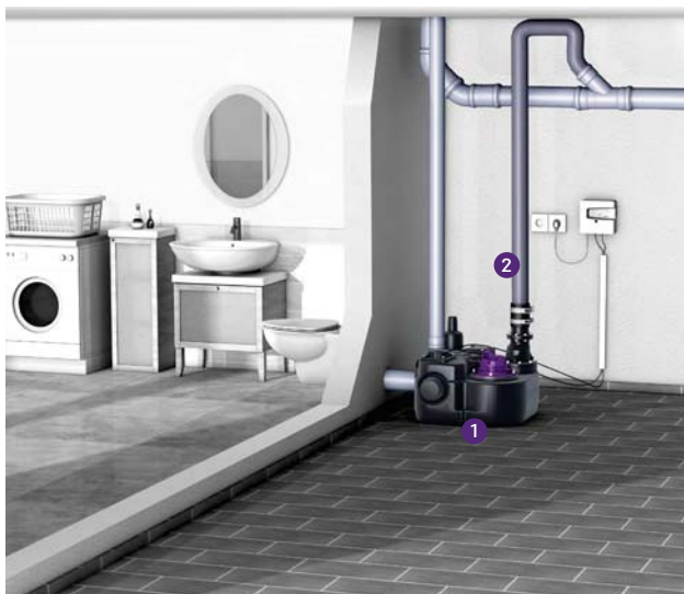
1 Lifting station 2 Pressure pipe
