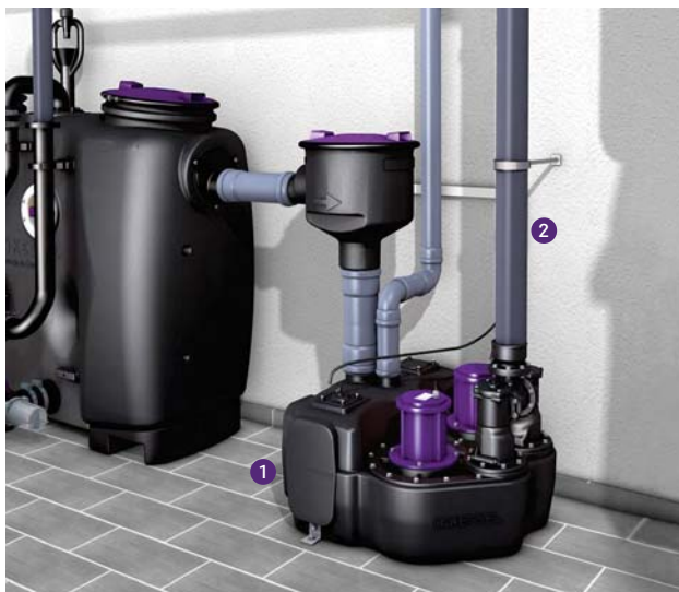
1 Lifting station 2 Pressure pipe
