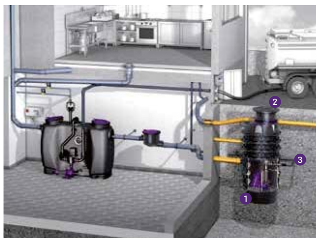
1 Pumping station 2 Engineering chamber 3 Pressure pipe
